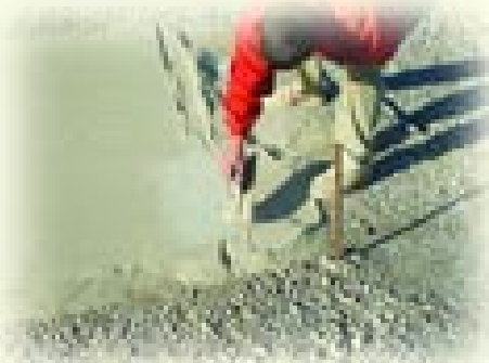
Filling the trough w/ a trowel
